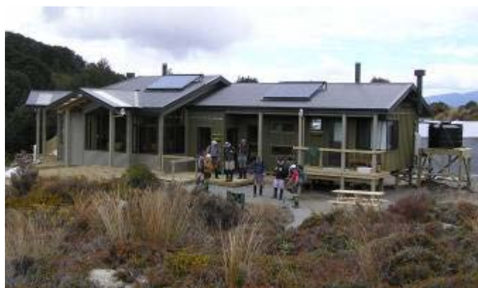
A new standard in DoC huts. 29 bunks with showers, solar lights & heating & great views of the peaks nearby. Decking not complete at time of trip. K.Fisher image
