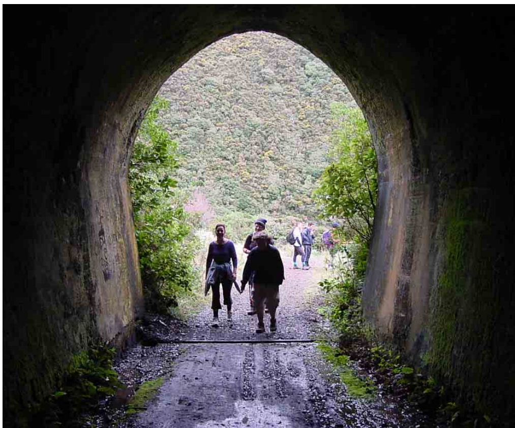
Above: One of the tunnels on the Rimutaka Incline (Photo: Tim Swale).
